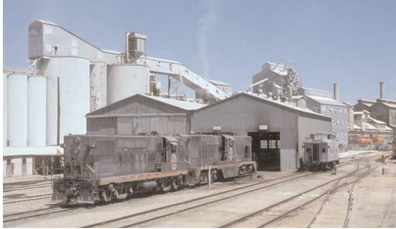
Trona's Baldwin's await the next run in front of the four bay diesel shop. Selective compression can be used to model this structure into a two bay diesel shop on the layout.
